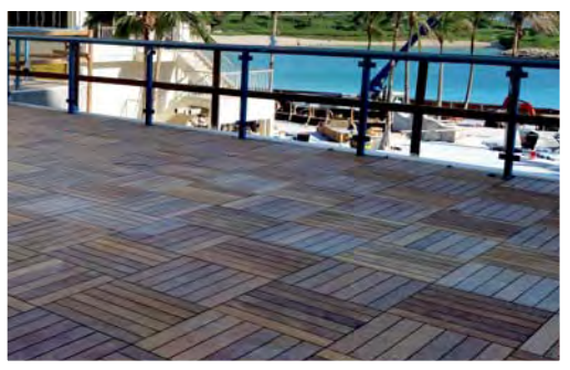
Honolulu Roofing installed Ipe pavers on the Kohala Deck at the Four Seasons Resort Oahu at Ko Olina.
