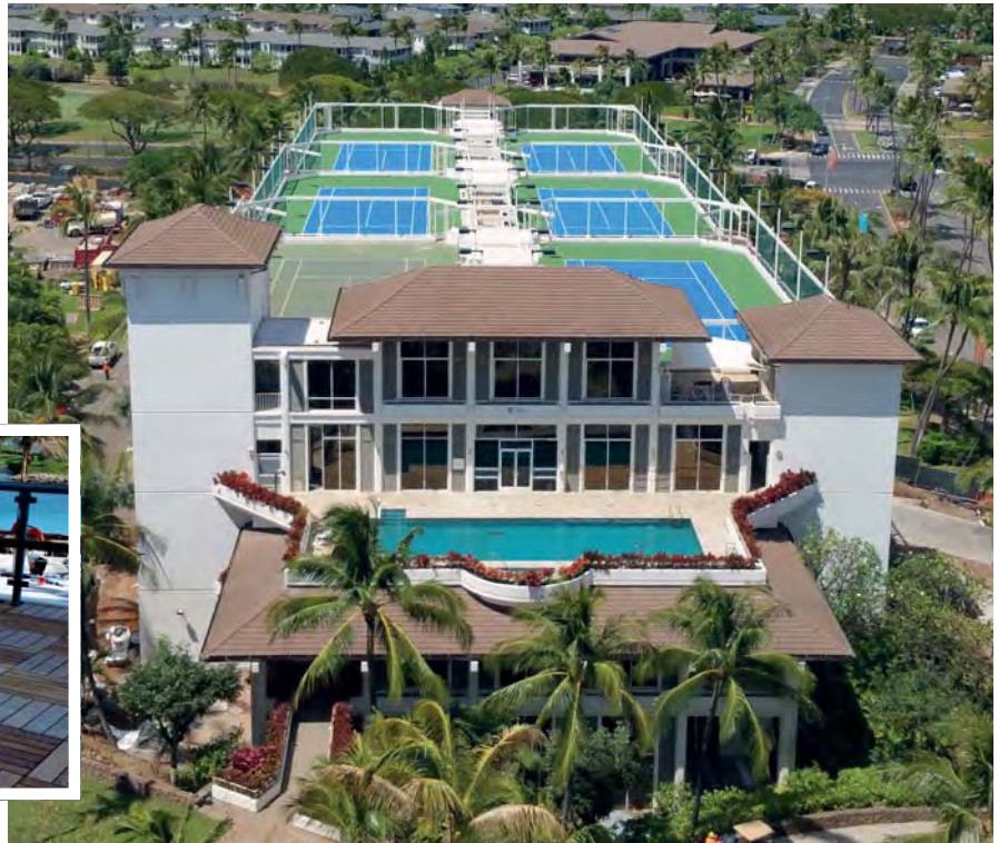
Honolulu Roofing applied Plexipave surfacing to the tennis courts at the Four Seasons Resort Oahu at Ko Olina.
